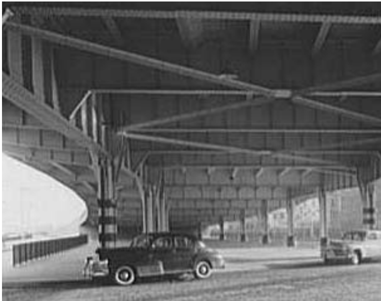
Elevated FDR Drive
